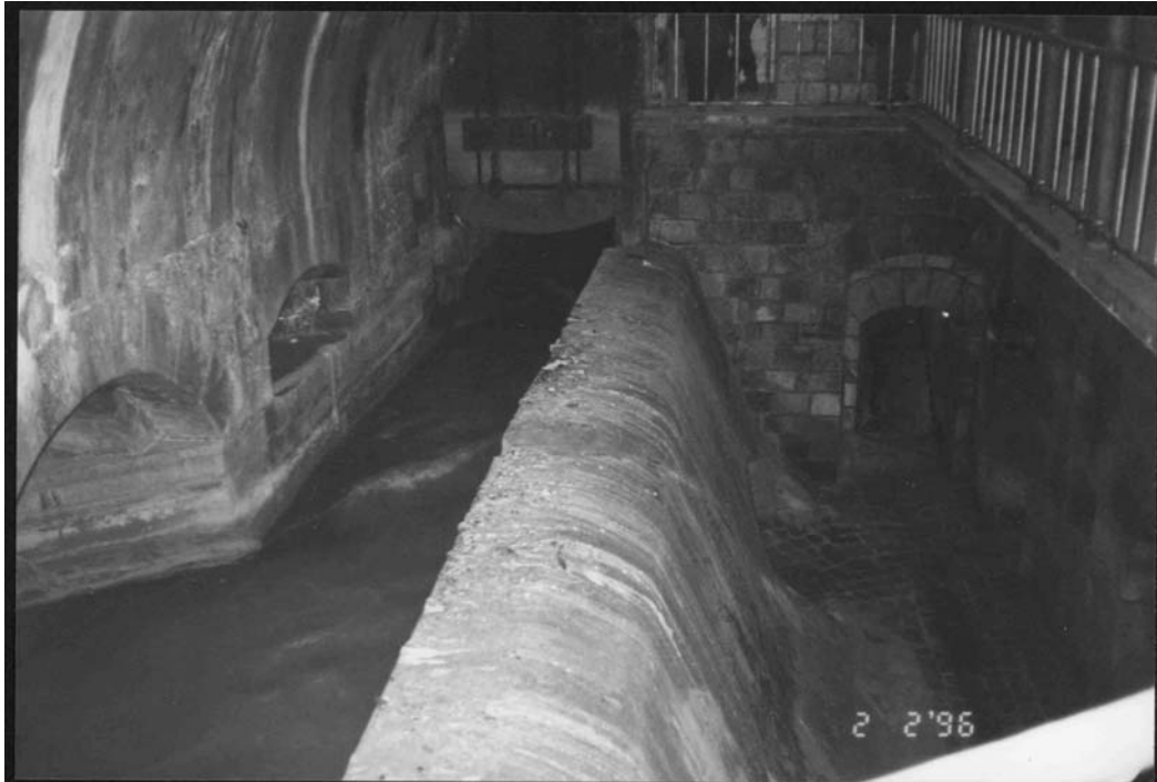
Figure 2: Overflow structure in the sewer network of Vienna (Austria). If the combined wastewater sewer at the left side of the picture is brim-full with the mixture of sewage and stormwater the excessive volume gets discharged directly to the Danube river by overflowing the dividing wall in the middle of the picture. The residues on the wall coping show that it is waste water which gets discharged and not rain water, even though this phenomenon is often called “stormwater overflow” in the literature.
