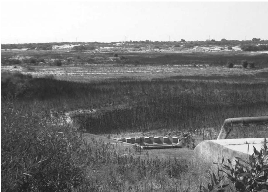
Figure 2: Infiltration basin of Menashe Artificial Recharge Plant, Israel, with intake building in the foreground (Gutman 2007)
