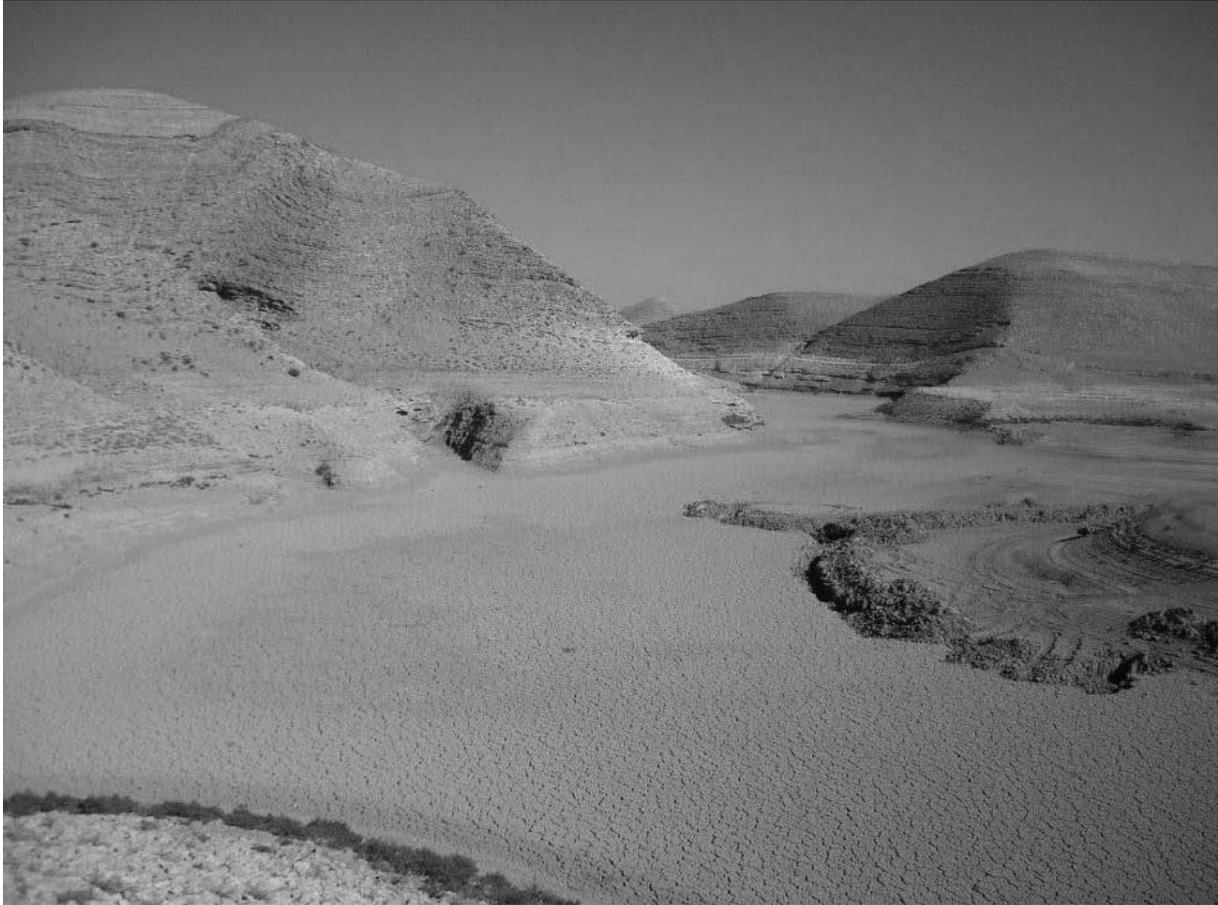
Figure 4: Bottom of the WALA Infiltration Reservoir, Jordan, covered with several meter thick silt and clays from four flood events. The sediments strongly reduce the original infiltration capacity of the reservoir.
