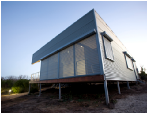
Fig. 14: The Hollingworth House – with the perforated fire shutters down at dusk. [Photograph by Andrew Halsall 2008]
