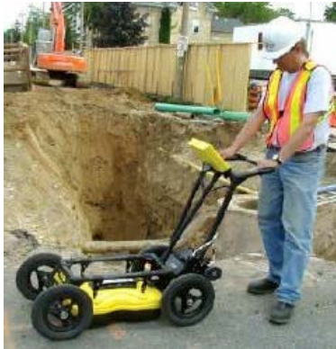
Ground Penetrating Radar
